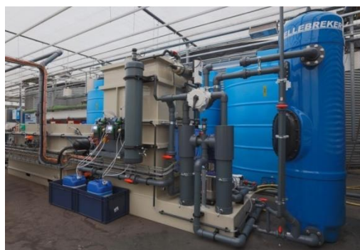
Figure 3-11. An example of a pilot installation for electrophysical precipitation in a horticultural greenhouse
