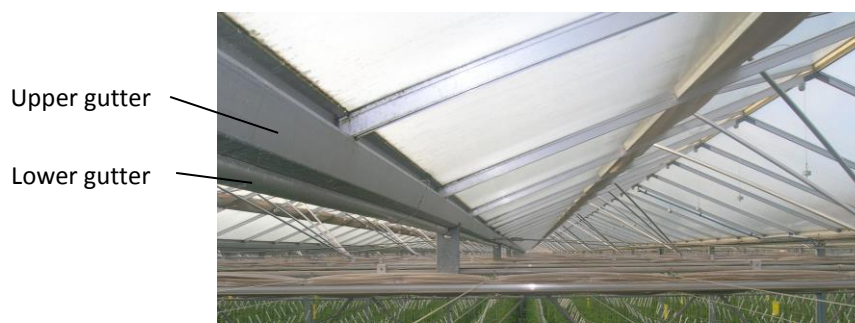
Figure 2-40. Picture of Venlo-type greenhouse with a double gutter for condensed water collection (Source: Santiago Bonachela)
