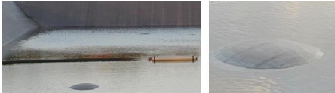
Figure 2-3. Bubbles indicate the presence of water or air underneath the foil. In case bigger bubbles are formed, this can lead to the rupture of the foil. Water underneath the foil also can harm the dikes (Source: PSKW)
