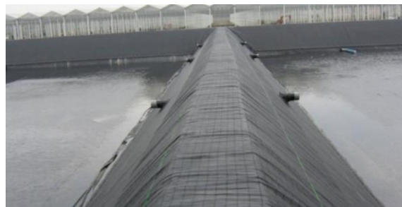
Figure 2-8. Intermediate dike separating 2 water reservoirs to avoid billow
