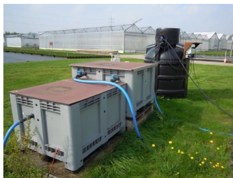
Figure 12-8. MBBR at PCS (Belgium)
