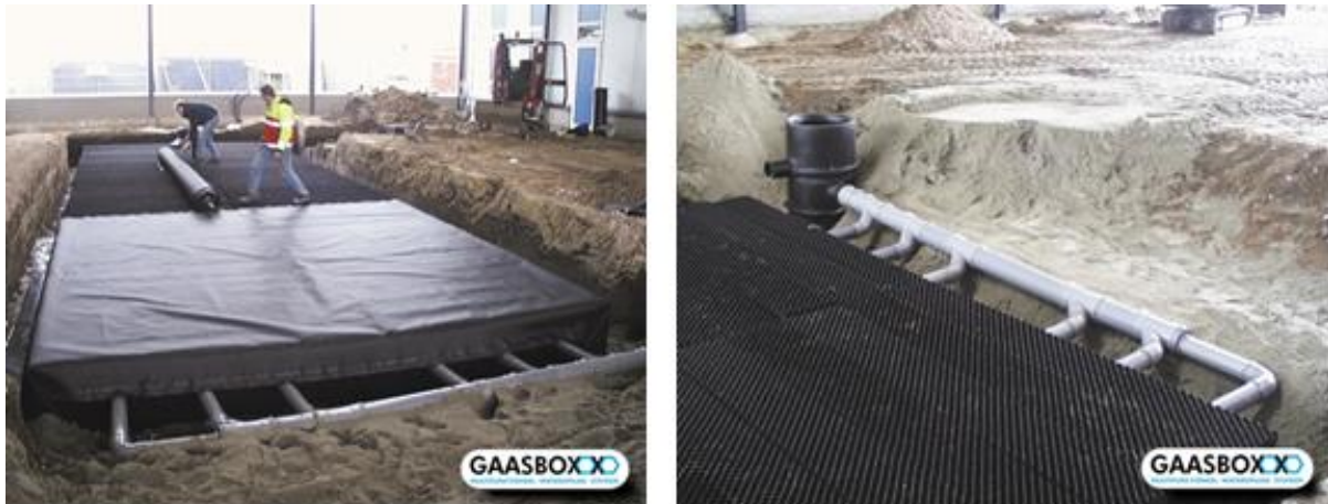
Figure 2-14. Installation of Gaasboxx ( https://jesproducts.nl/gaasboxx-systeem.htm )
