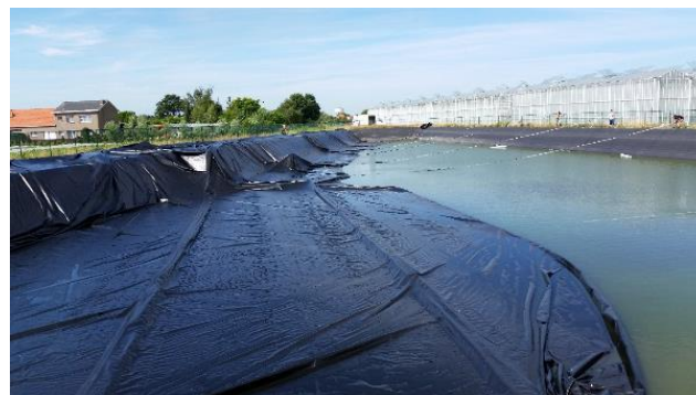
Figure 2-33. Manpower is needed to put the foil in its final position, so installation takes some hours (Source: PSKW)
