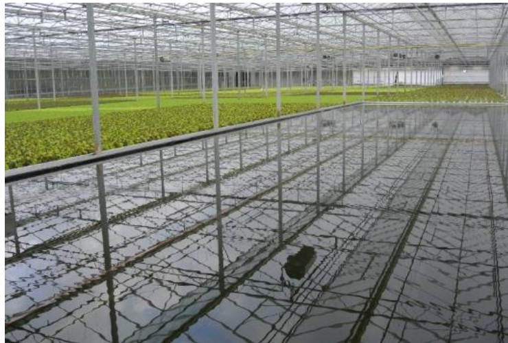
Figure 9-16. Deep flow installation
